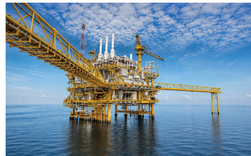
Figure 2. An ExxonMobil deepwater oil and gas facility.
